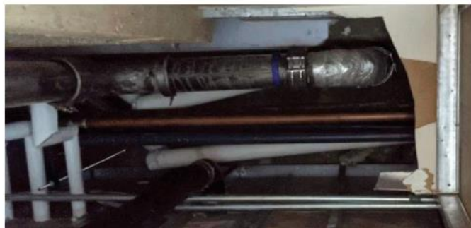
Images: Portions of broken acid waste piping and piping repairs in shaft utilizing cast iron instead of glass.
