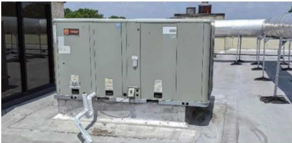
Images: Commonly observed original air-handling unit with compromised supply duct insulation.
