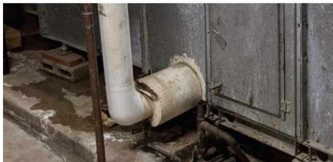
Images: Gas-fired domestic hot water heater next to the heating water boilers with uninsulated domestic hot water piping.
