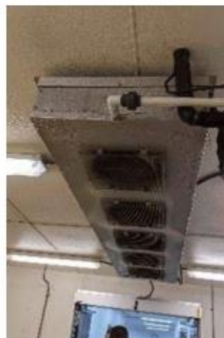
Images: Supplemental cooling unit for instrumentation lab with portable cooler. Walk-in cooler condensation resulting from adjacency to tempered loading area.
