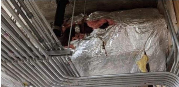
Images: Commonly observed original air-handling unit with compromised supply duct insulation.
